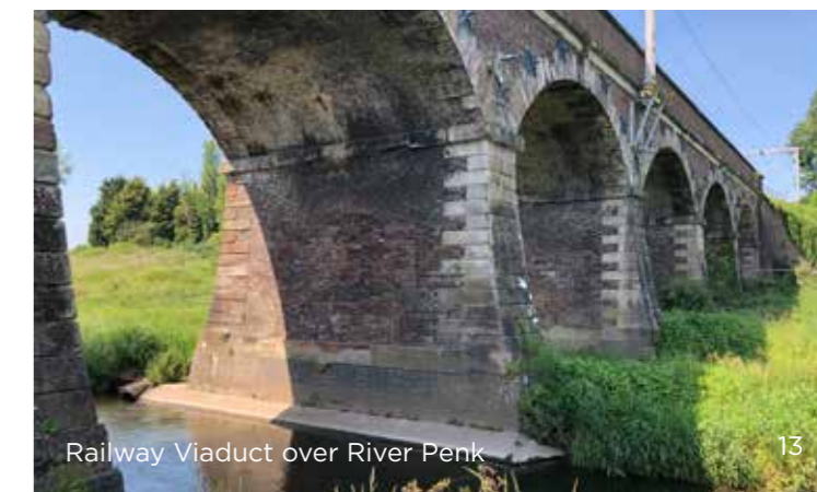
Cuttlestone Bridge (Listed)
